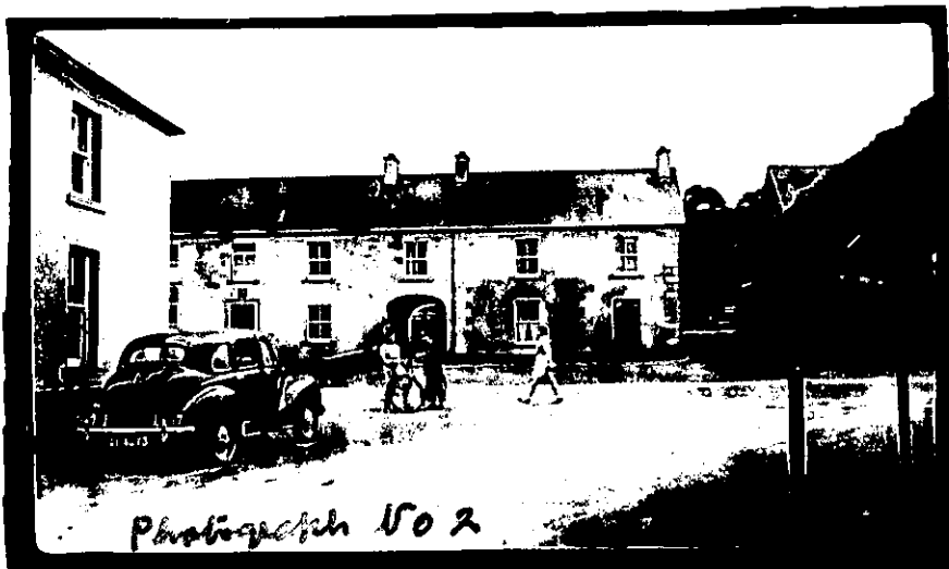
Photograph No. 2: Another view of the barrack and Mitchel's lock-up store. On the right of this photograph can be seen a portion of a lean-to shed attached to Mitchel's shop - No. 1 post - on the opposite side of the road from the barrack.
